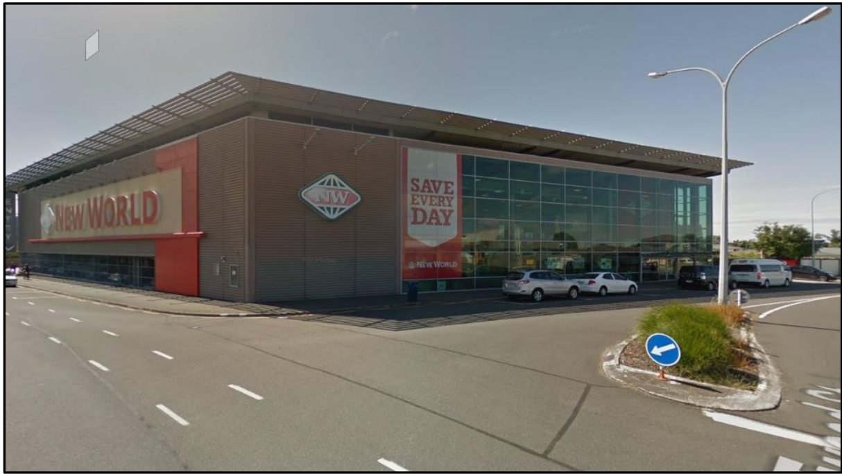
Figure 3- Reference Image of Supermarket Facade
